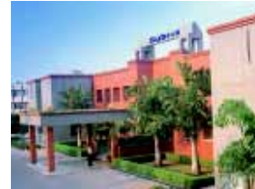
Noida Central Plant
